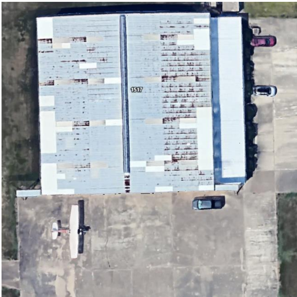
Overview of Hangar at Sugarland Regional Airport
