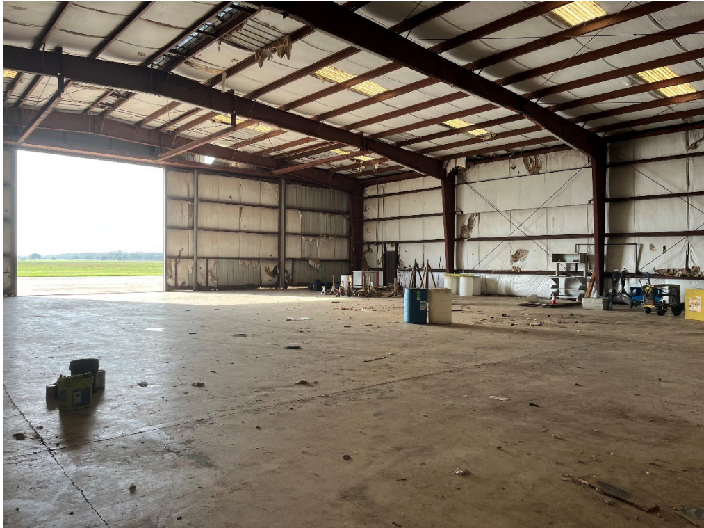
Additional Picture of Hangar
