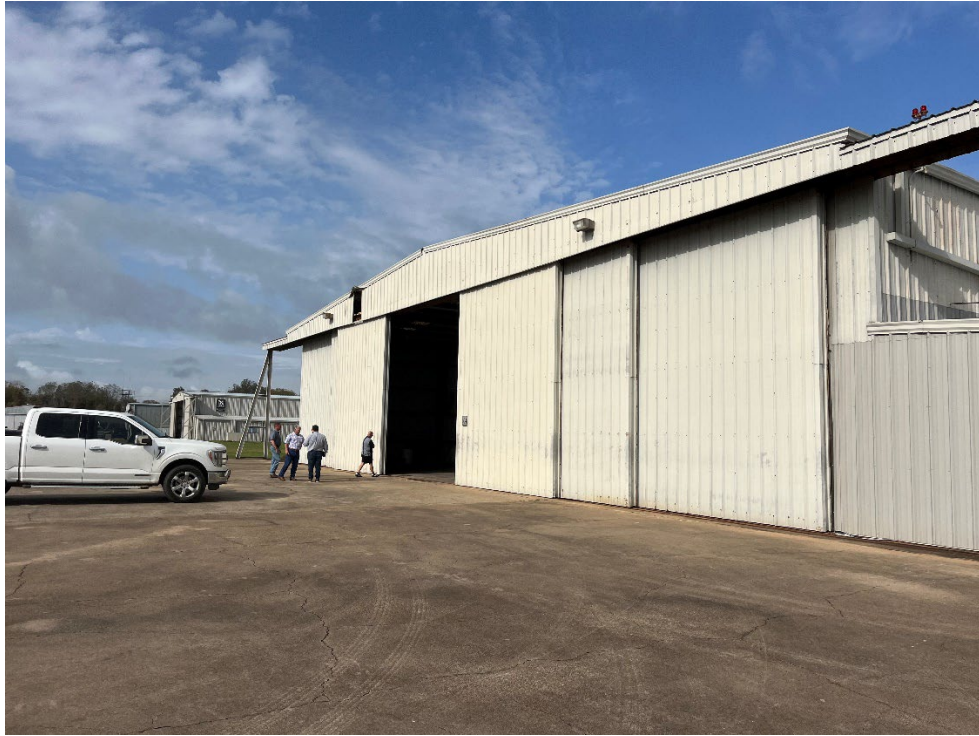
Additional Picture of Hangar
