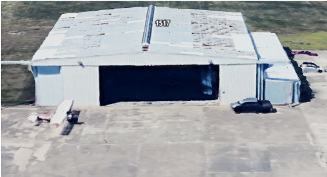
Front View of Hangar at Sugarland Regional Airport
