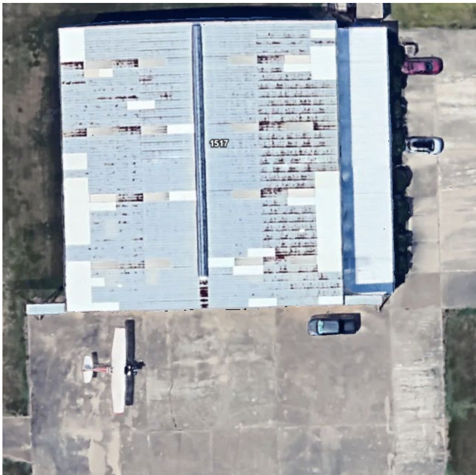
Overview of Hangar at Sugarland Regional Airport
