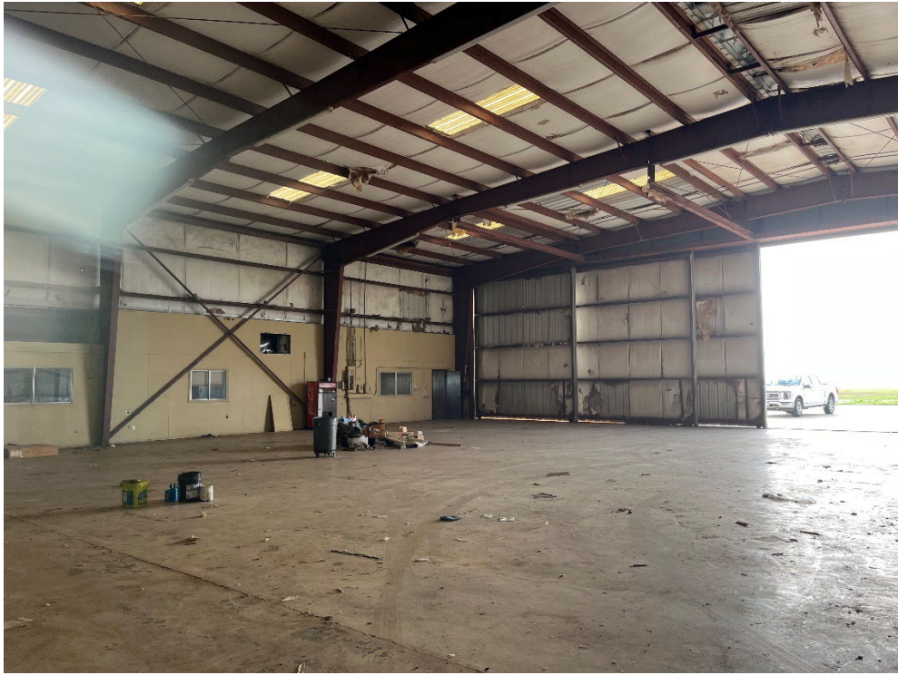
Additional Picture of Hangar
